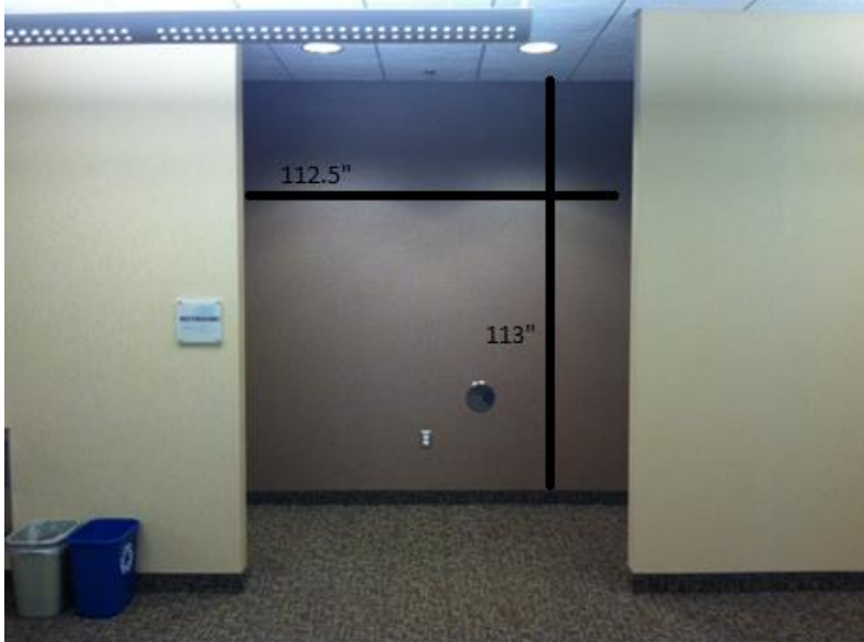
Location 6: 1 st Floor Gallery – South Wall between Restrooms
