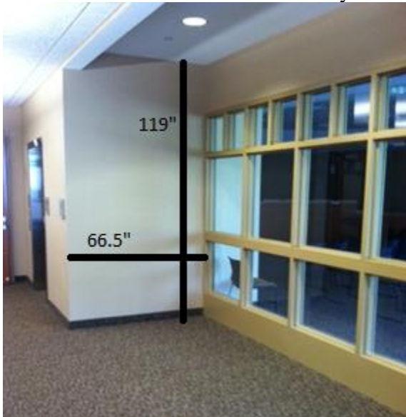
Location 7: 1 st Floor Council Hallway – Western Wall
