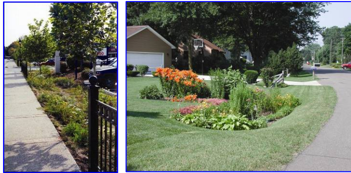
Figure ES-2: Rainwater Gardens Designed to Treat Impervious Area Runoff
